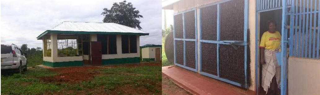
PHOTO 1 (a): Evaporative Charcoal coolers in Makueni, Kenya PHOTO 1 (b): Front view of such a cooler
